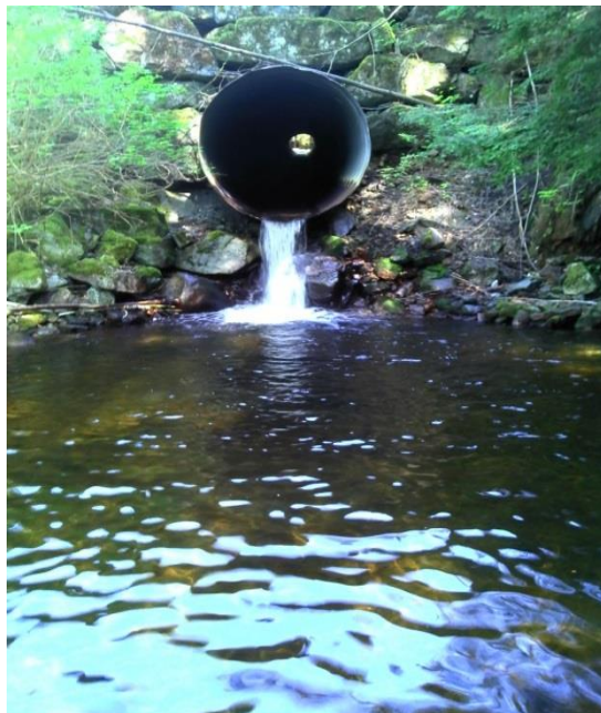
Figure 1.–Hoadley Creek barrier culvert.
