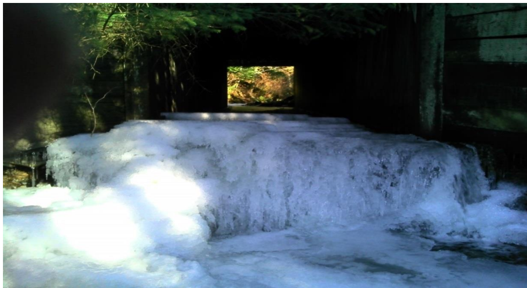
Figure 1.–101-47-10300 culvert barrier in the winter.
