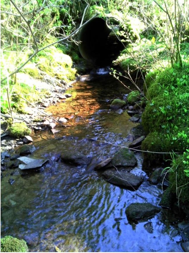
Figure 1.–Culvert crossing on 101-47-10145.
