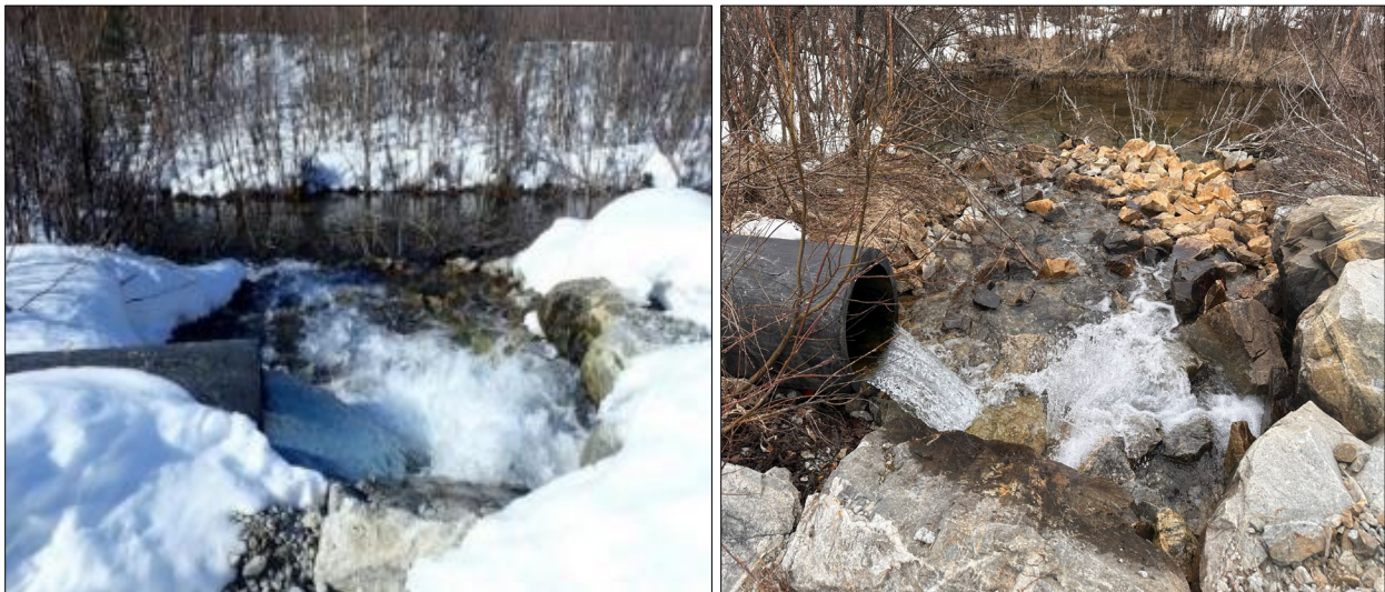
Figure 4.—Outfall 002 RO water discharge: up to 3,000 gpm during 2019–2021 (2020 left) and reduced to approximately 400 gpm during 2022–2025 (2025 right) into the RO Channel wetlands.
